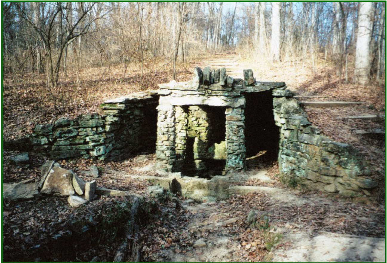
The springhouse over Red Bud Springs, built by Joseph Griesedieck of Falstaff Brewing, is just one scenic ruin present in the park.
